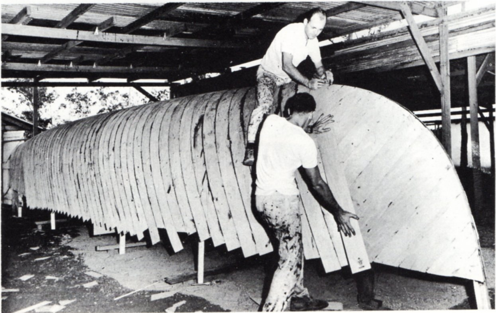
MOULDED PLYWOOD HULL BEING BUILT AT MARINE PARK.
