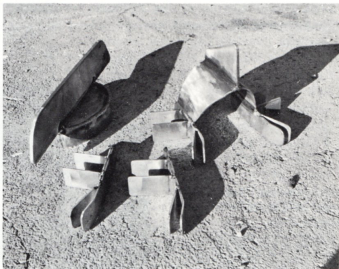
Mast fittings may be home made or at least made by local metal shop.
